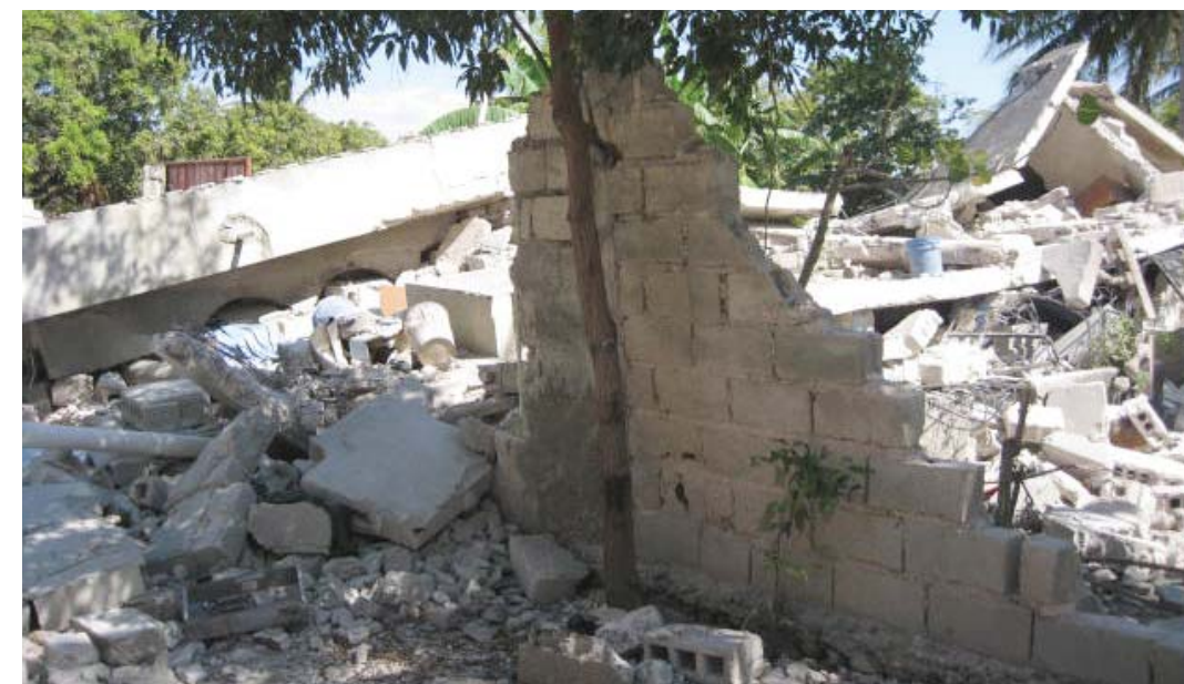
Collapsed building behind the orphanage in Haiti
